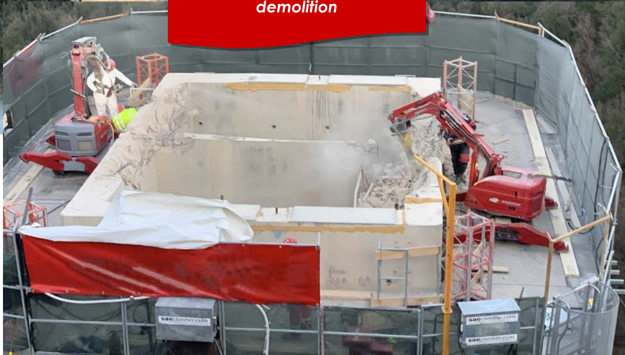
Pluri Mast for highway piles demolition
