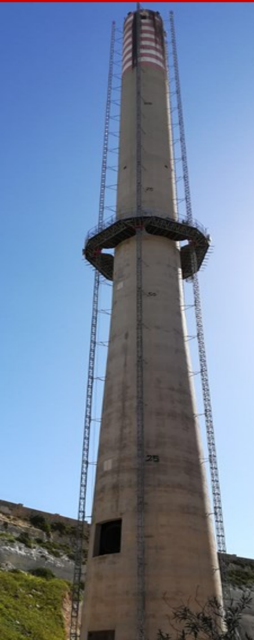
5 mast chimney demolition with service hoist
