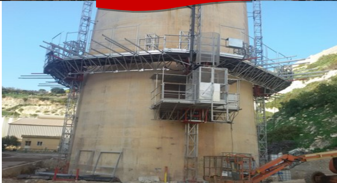
5 mast chimney demolition with service hoist
